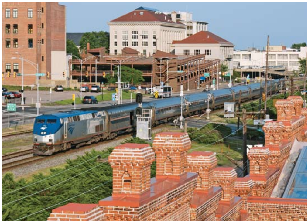
ABOVE: The southbound Carolinian is seen passing the historic tobacco warehouses of downtown Durham. The city once boasted a grand Union Station which served five railroads in its heyday, but it was demolished in 1968 to make way for a new road and parking garage (visible in the distance). The brick structure in the foreground is the restored Walker Warehouse, as of June 2009 the site of Durham's new Amtrak station. NICHOLAS D'AMATO
